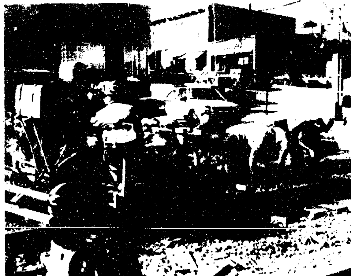
SECURING THE TRACK WITH ANCHORS are Conrail men Roger Cooper and Sammie Hill, at far right in the photo. The men were working near the Main St. railroad crossing in Chelsea. Ad-
