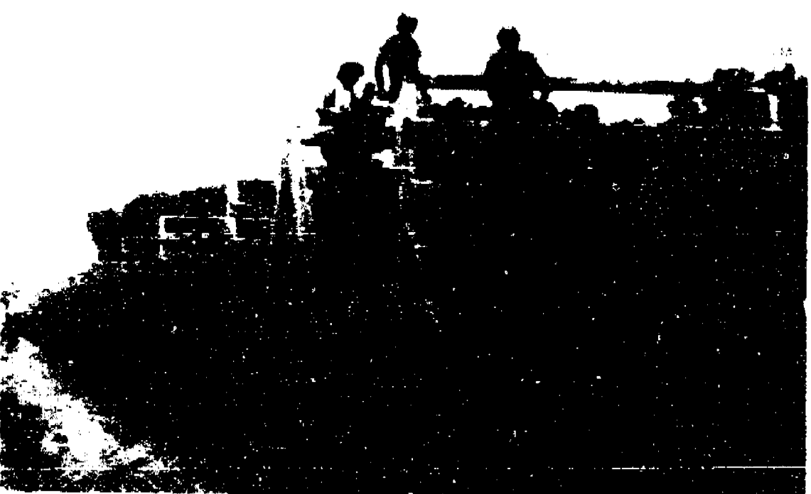
WELDED RAIL COMES IN 1,300-foot lengths and is transported on a special train that stretches a quarter-mile. Here, three workers have used sledgehammers to break off anchors and allow
