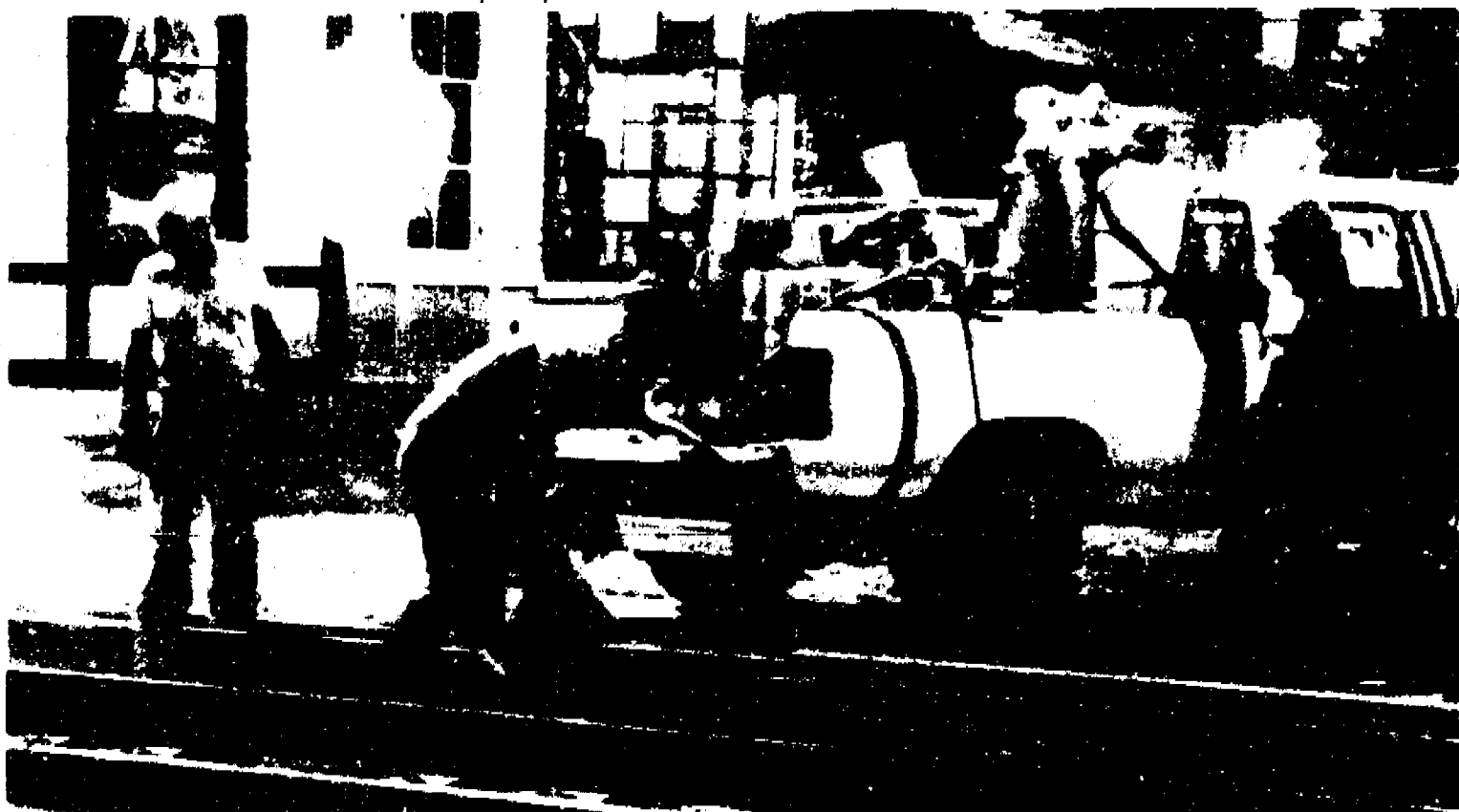
A CARBIDE SAW is used by Conrail workmen to cut into a length of track. The men did this work on one of the 50 degree days last week. Sections of the rail, ranging from 1,300 feet to 1 1/2 miles are
